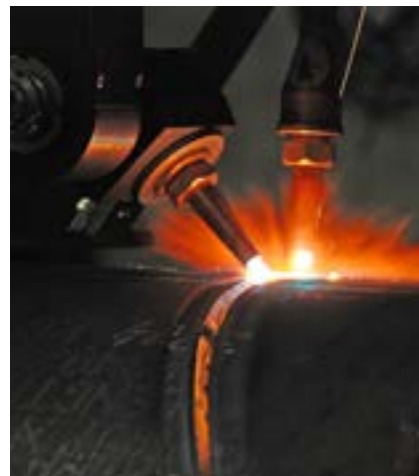
Pre-heating during cutting
