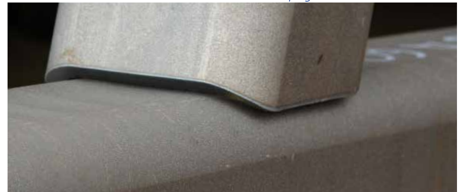
Box section saddle connection
