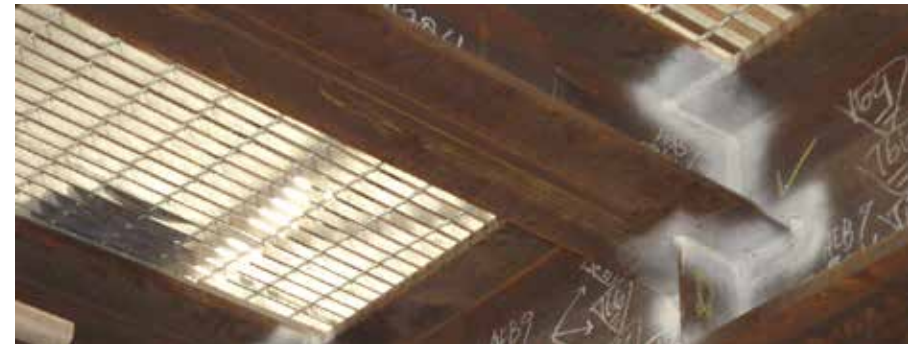
Fitting and welding in detail
