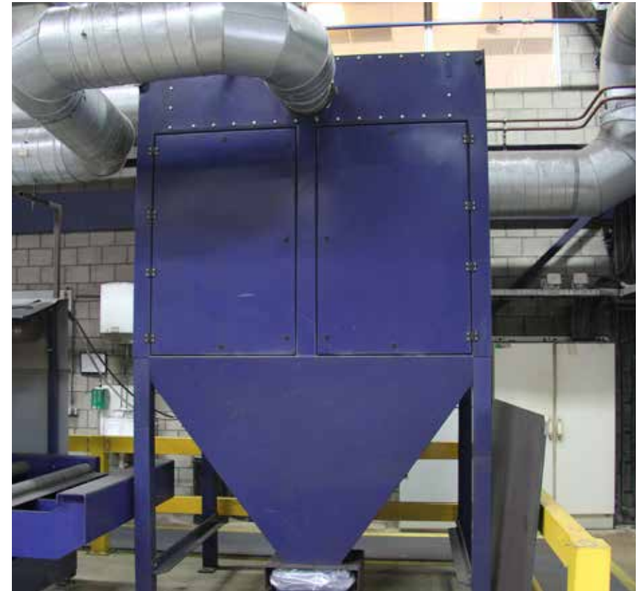
Fume extraction unit and particle filter
